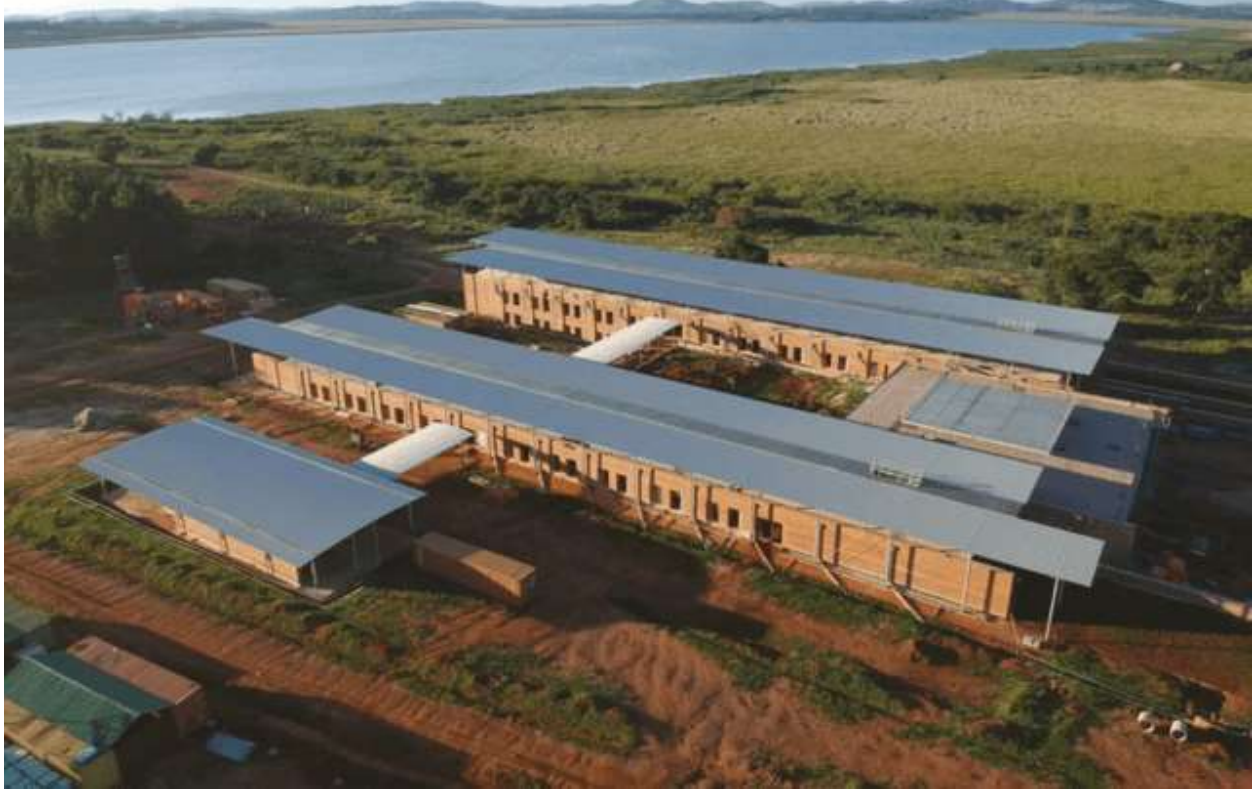
Fig. 2: Renzo Piano completes Uganda Children's Hospital with Stabilized earth walls. Image source: [4]
